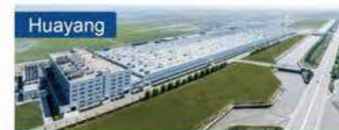
Huayang Passenger Car Radial (PCR) & Light Truck Radial (LTR) 8 million units
